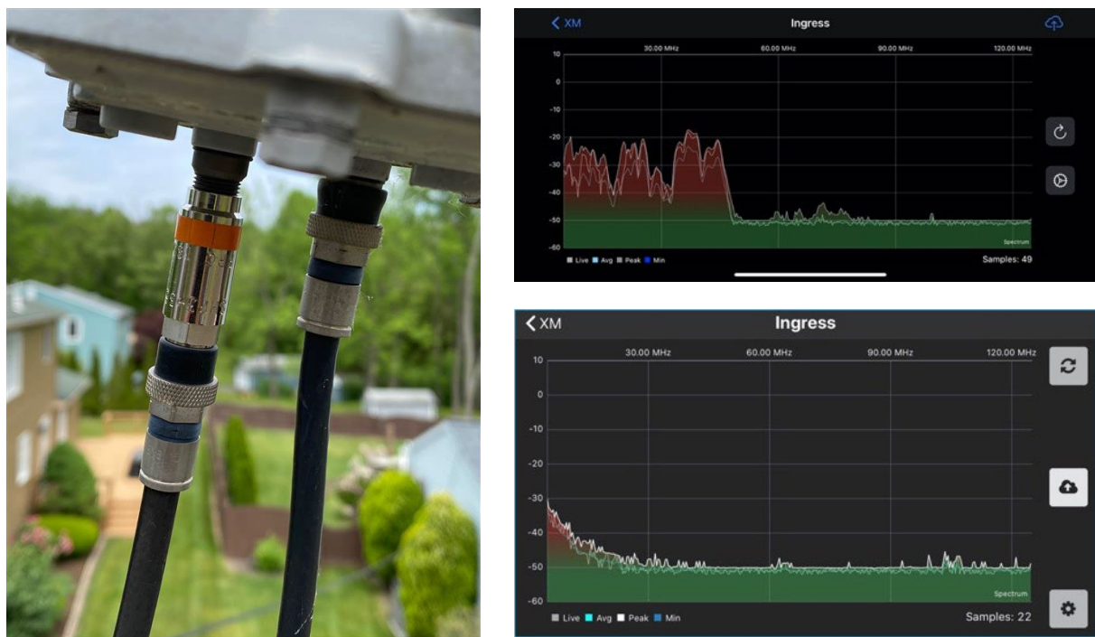
Figure 25 – Noise trap / filter (left), before (top right) and after (bottom right)
