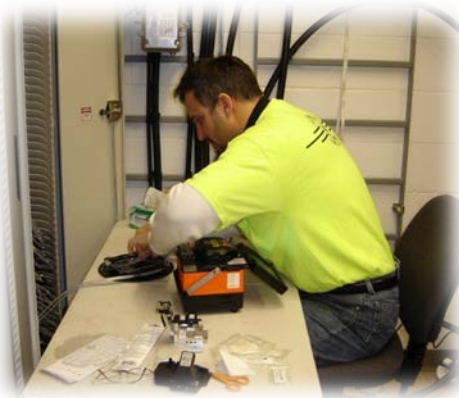
Figure 2 - Fusion Splicing (as described above)
